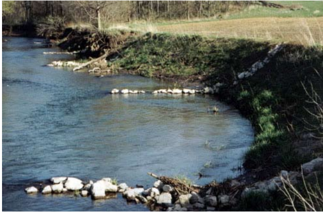
Figure TS14H-3 Bendway weir (Photo courtesy of Wayne Kinney, NRCS)
