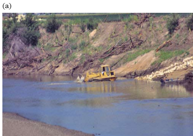
Figure TS14H-2 (a) Bendway weir, under construction; (b) Completed bendway weir (Photos courtesy of Mark Locke, NRCS)
