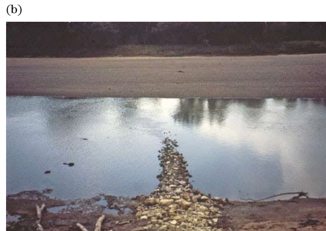
Figure TS14H-2 (a) Bendway weir, under construction; (b) Completed bendway weir (Photos courtesy of Mark Locke, NRCS)
