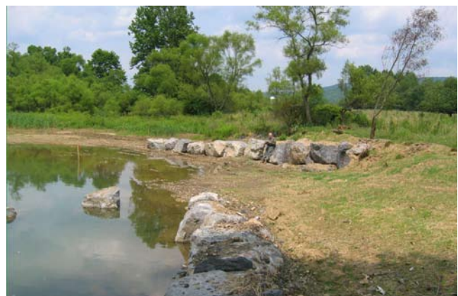
Figure TS14H-6 Rock vane
